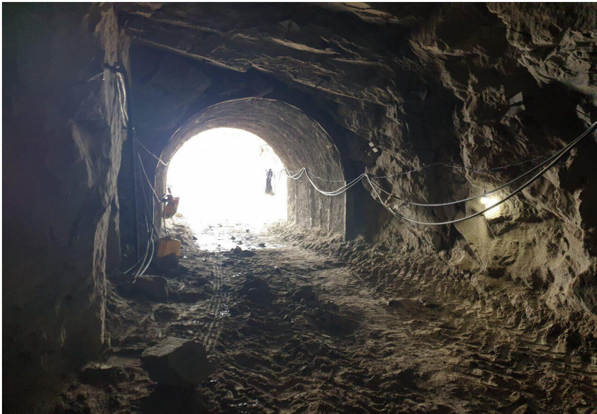
Fig.2 Tunnel Portal under construction.
