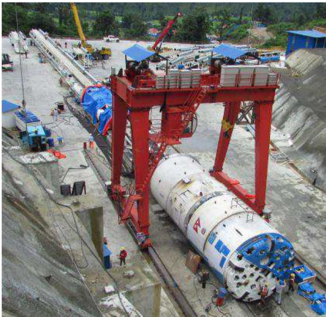
Fig 9.1 Showing the TBM in Bheri Babai Project
